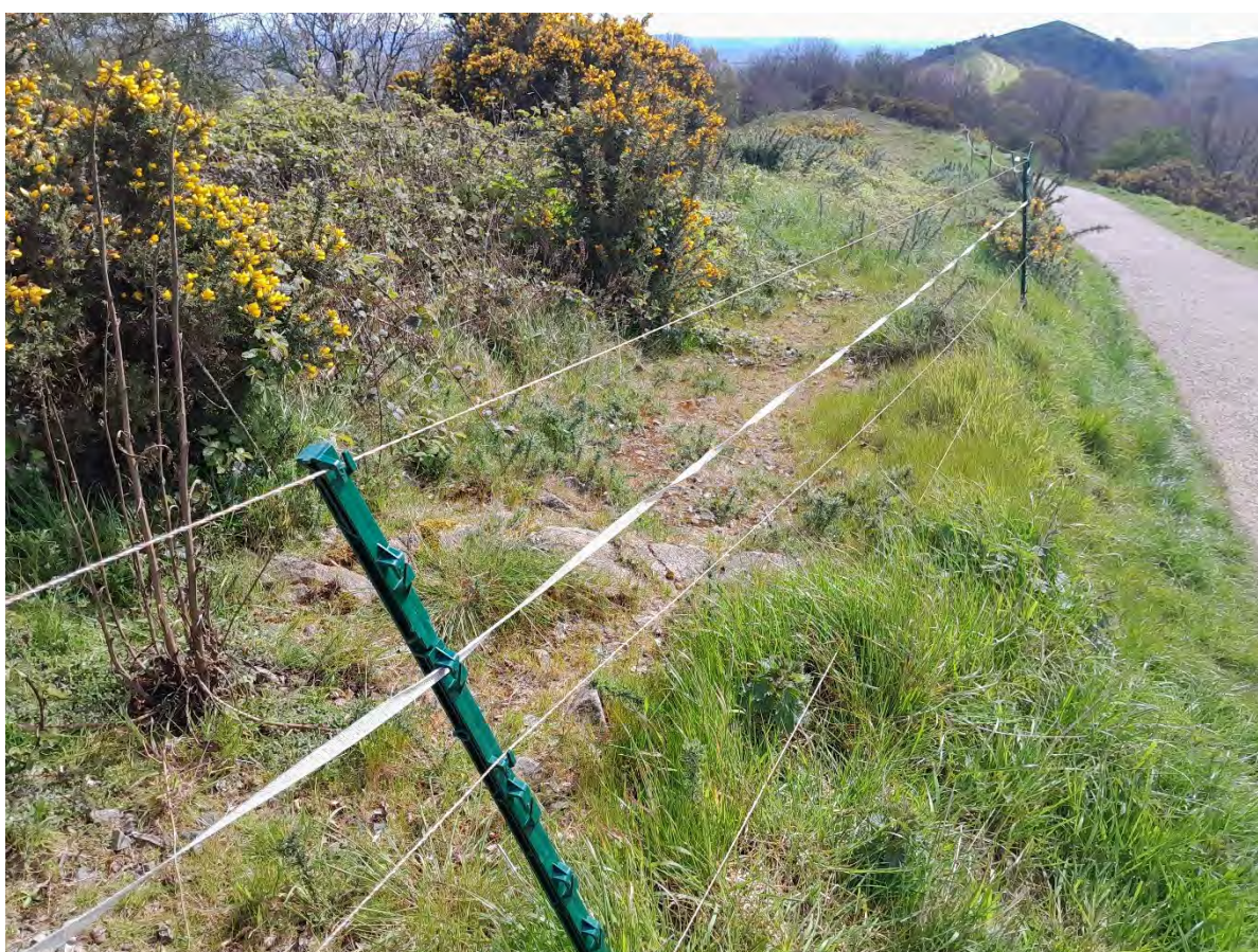
Restoration of an eroded area, Beacon Road
