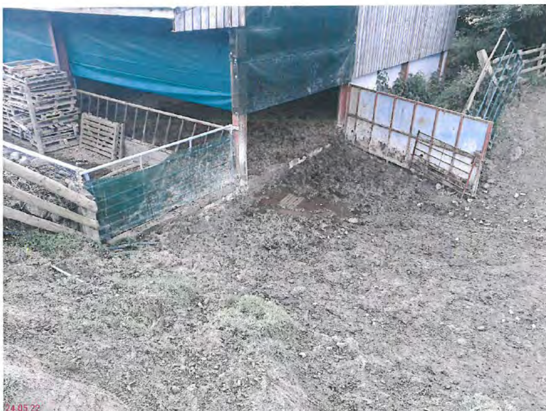
Photo 2: existing entrance to shed
