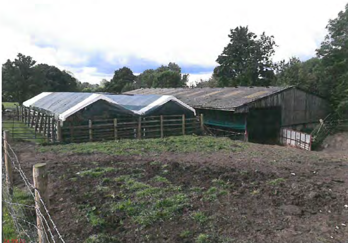
Photo 1: Tarpaulin structure (left) adjacent to existing agricultural shed.
